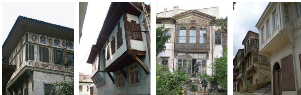
Figure 11-12-13-14: Examples of Ottoman Houses ( Birgi Çakırağa Mansion, Kütahya Houses, Muğla Karaosmanoğlu Mansion, Trilye-Bursa Houses ) Photographed by Hayriye Oya Saf
